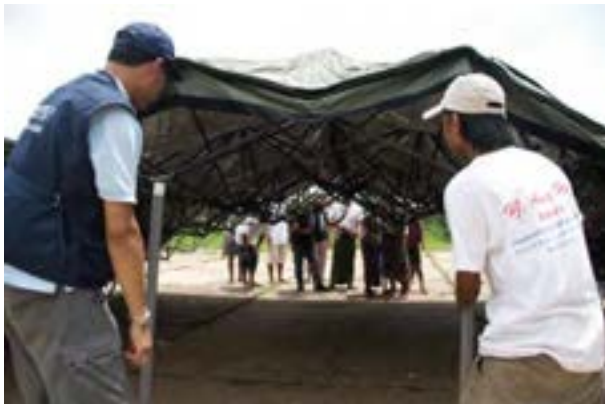
Only 4 men was required to deploy the 30sqm system shelter.
